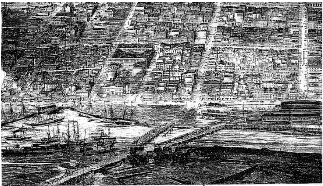
Turning Basin / Port of Melbourne Falls Bridge Railway Bridge
